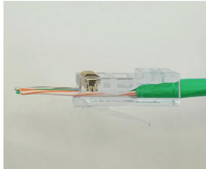
Push the plug as far down onto the cable until it stops inside the plug.
