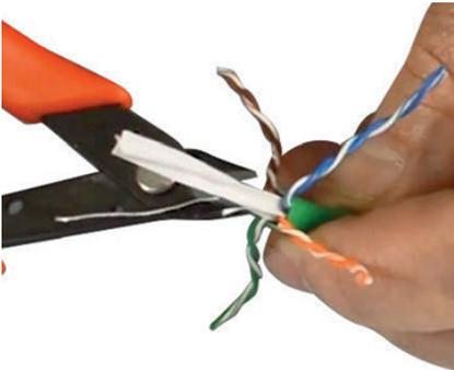
Trim center spline/pair separator as close to the cable jacket as possible without nicking any of the wire conductors.
